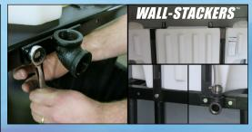
Bolt elbow to the stand's centermost pre-drilled holes.
